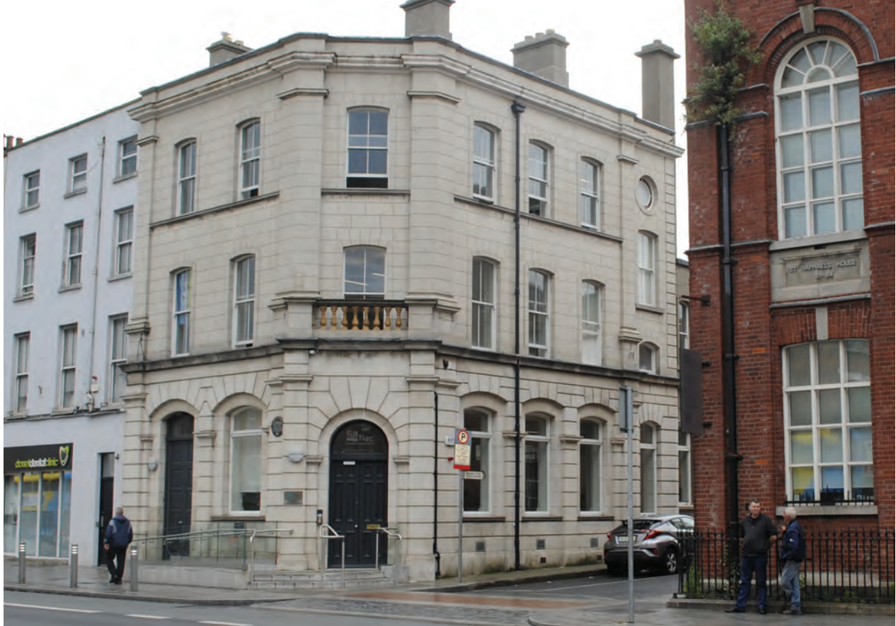
FLAC's Offices at 85/86 Dorset Street Upper.
